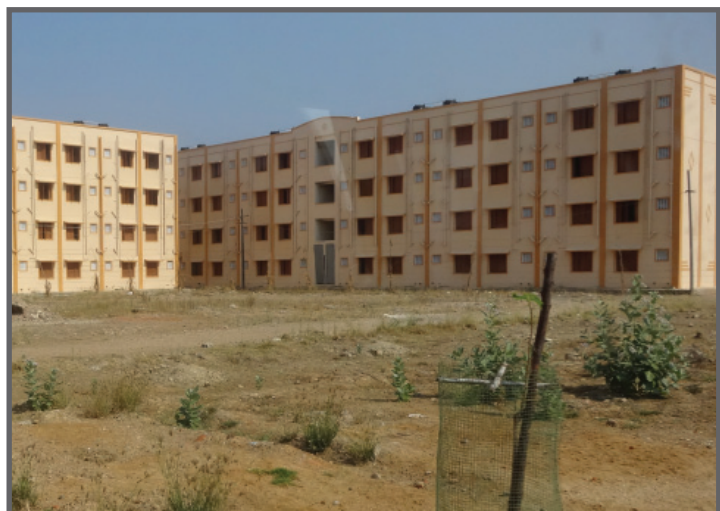
ETRP POST-TSUNAMI HOUSING IN EZHIL NAGAR, CHENNAI
