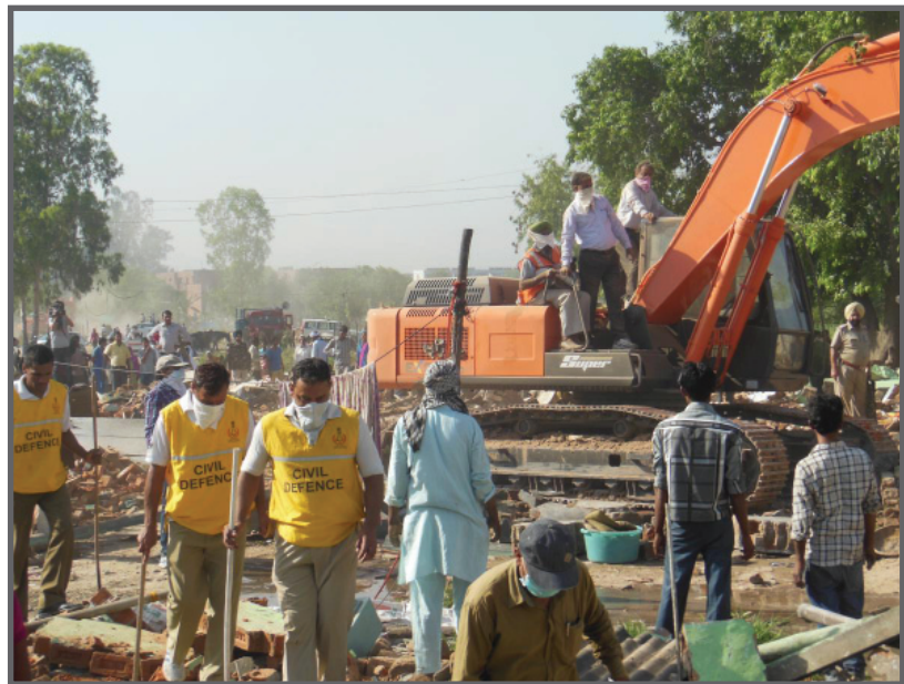
DEMOLITION IN CHANDIGARH
