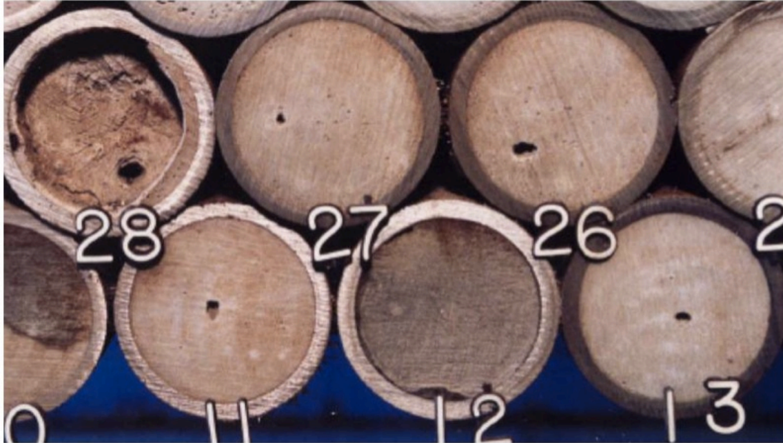
Figure 11: Channels and gas pockets caused by faulty cementing are a possible channel for contamination. Source: Watson 2004, quoted in Dusseault 2014.
