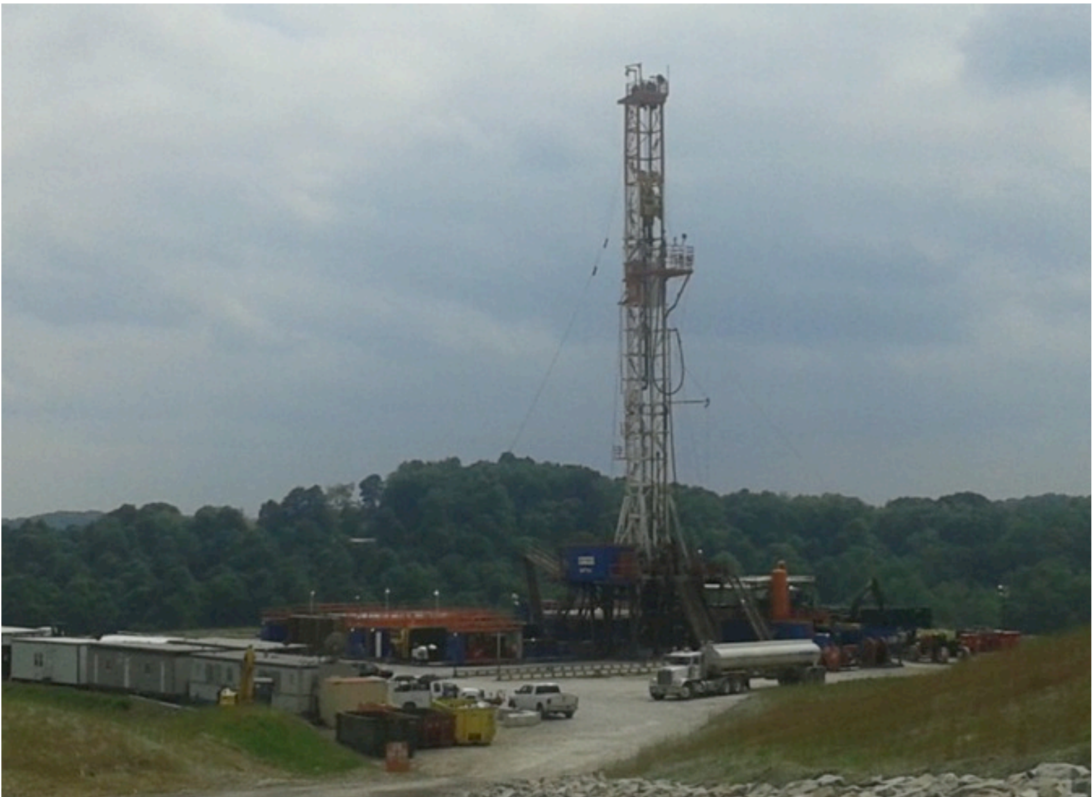
Figure 1: Fracking drilling station near Pittsburgh Pennsylvania. Photo JDTaillant
