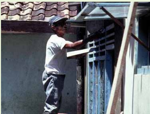
Shelter improvement by owners. Photo: Marc Jansen
