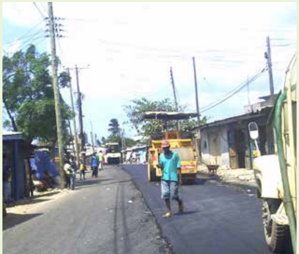
An inner neighborhood street being paved by CIUP
