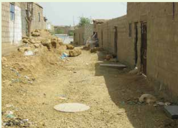
A recently completed lane sewer in Gulshan-e-Zia residential area, Orangi. Photo: Orangi Pilot Project.
