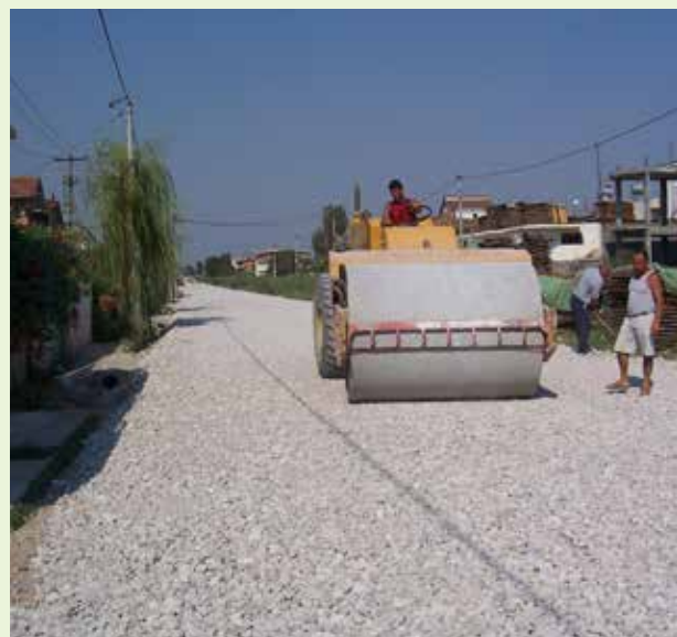
Residents organize themselves with support from the NGO CoPlan in the execution of their street plan using gravel pavement and compacting. A successful practice in the informal areas of Tirana, Albania . © Coplan.
