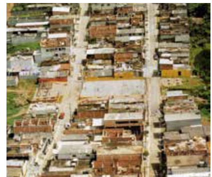
Illegal land subdivision in Sao Paulo, Brazil, showing regular street patterns. Photo: Municipality of Sao Paulo.
