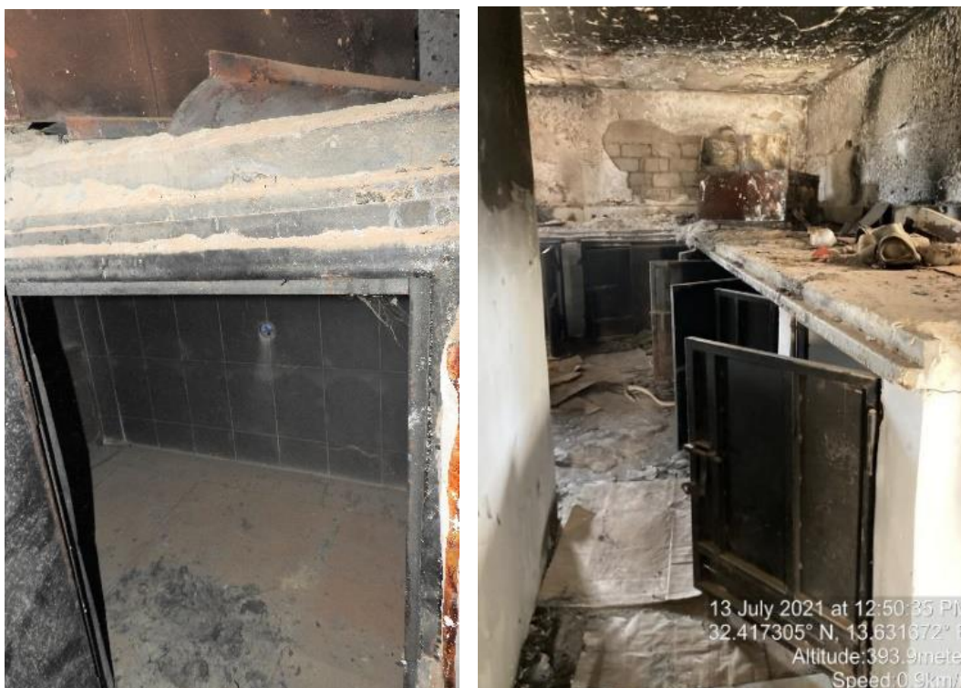
Photos taken by the Mission during site visits to the Boxes Prison showing the 0.8x0.8m boxes-like enclosures
