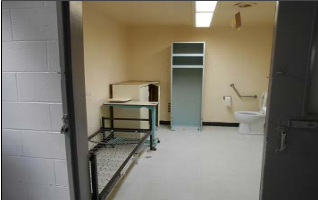
Federal Training Centre – Accessible cell
