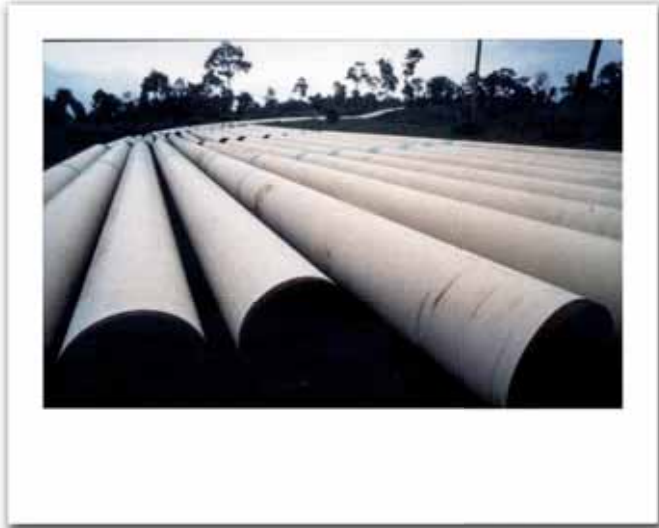
Yadana pipeline during construction © EarthRights International
