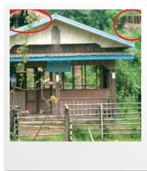
The same public health clinic in Zinba village, photo in 2009, showing two police barracks in the background constructed by local villagers with forced labor © EarthRights International, 2009
