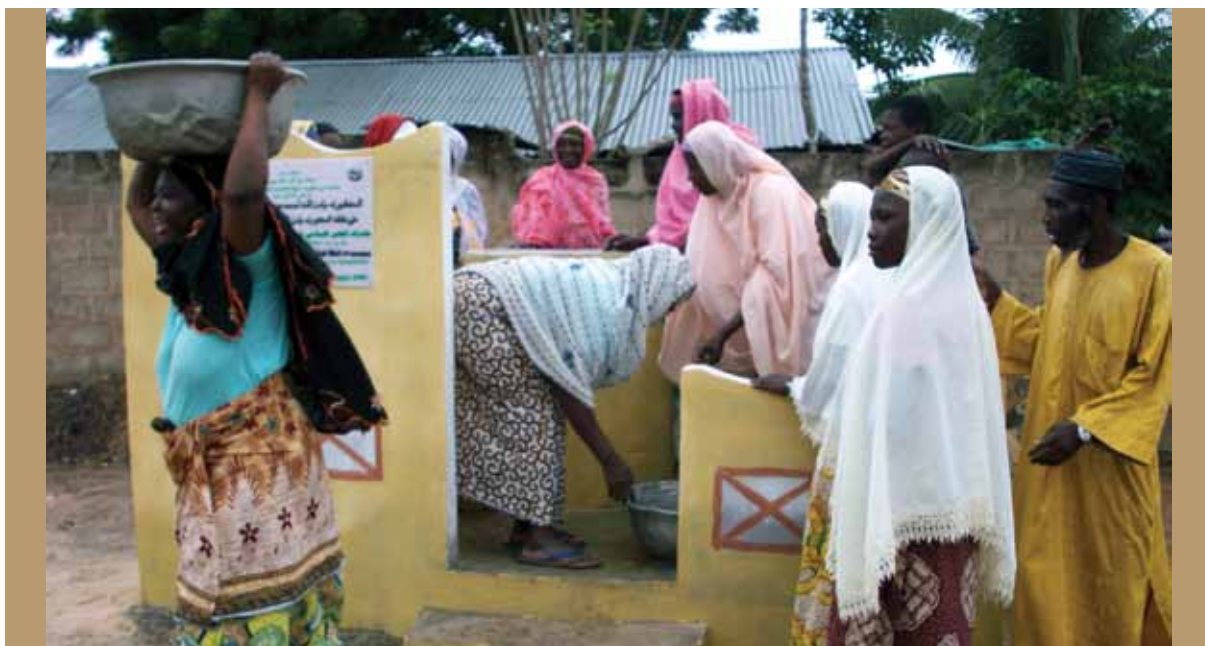
Dubai Charity Association financed the building of wells to provide the local community with clean drinking water in Benin.
